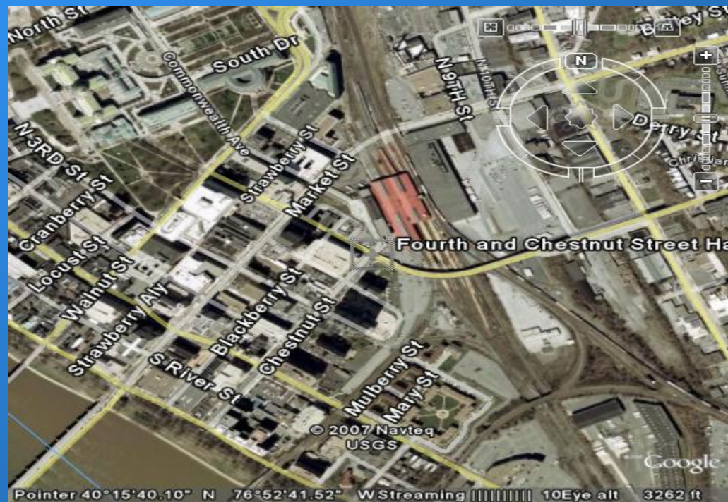
Figure VI.1 Aerial Photo of Harrisburg Amtrak Station
