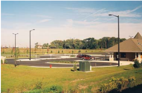
Figure VI.26 New Parking Lot at Sturtevant/Racine Amtrak Station
