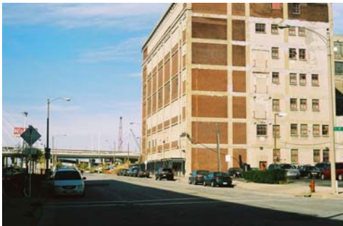
Figure VI.22 Commercial Office Building Across from Milwaukee Amtrak Terminal
